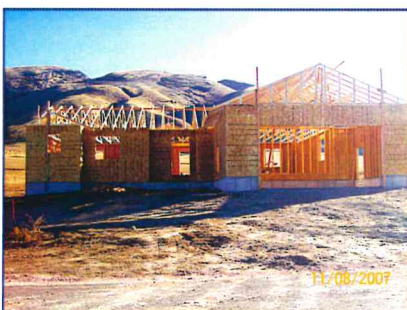
Montpelier home under construction, November 2007
