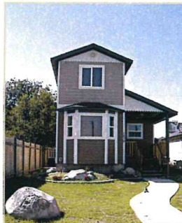
Completed home, front September 2009
