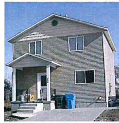
Completed Pocatello Home
