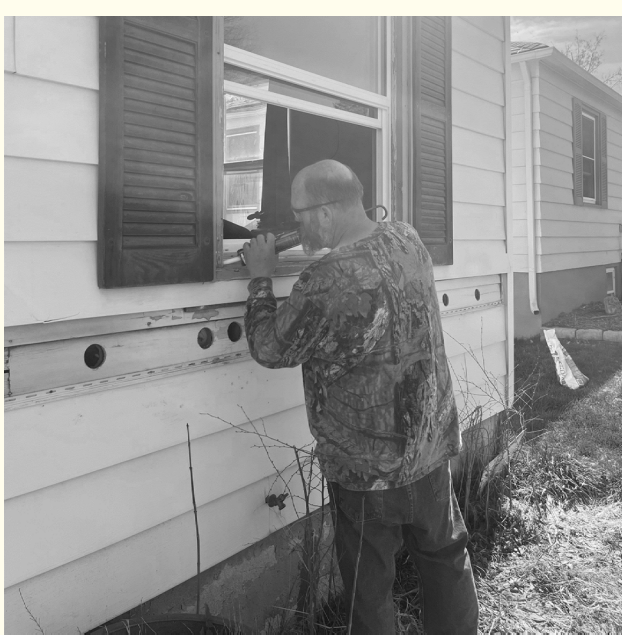
Mike Wilson caulking a newly installed window to prevent air leaks.
